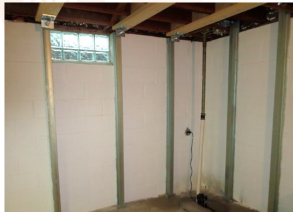
Photo 2. Beams with jacks.
