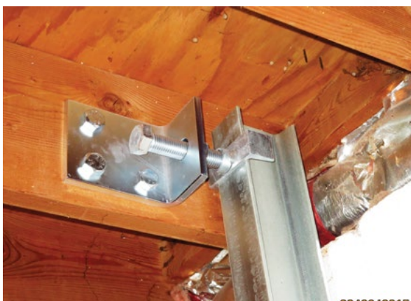
Photo 4. Jack on side of joist.
