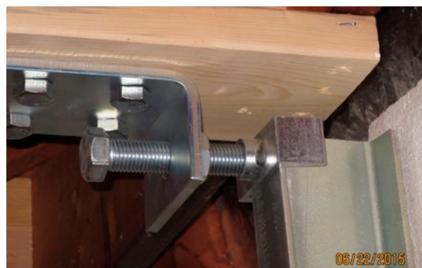
Photo 3. Jack at top of wall beam.
